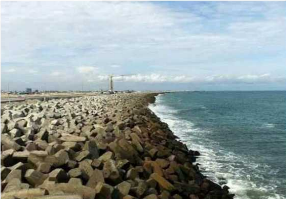
Coastal defense infrastructure by Lagos state government
