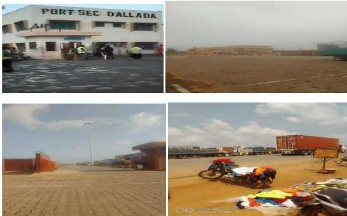
Photo 24: Dry port of Allada
