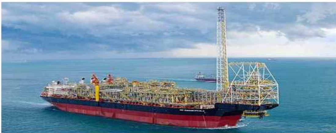
Fig. 12 FPSO John Evans Atta-Mills producing about 50,000 bpd
